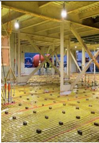
10.29.20 Vapor Barrier Area C Ready for SOG
