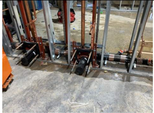
10.28.20 Bathroom Fixture Carriers C2
