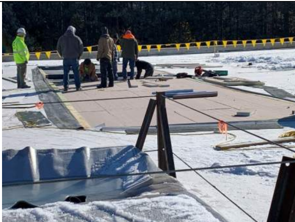
10.31 Saturday Roofing Crew Working on RTU Flashing
