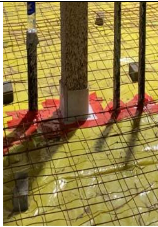
10.29.20 Vapor Barrier Area C Ready for SOG
