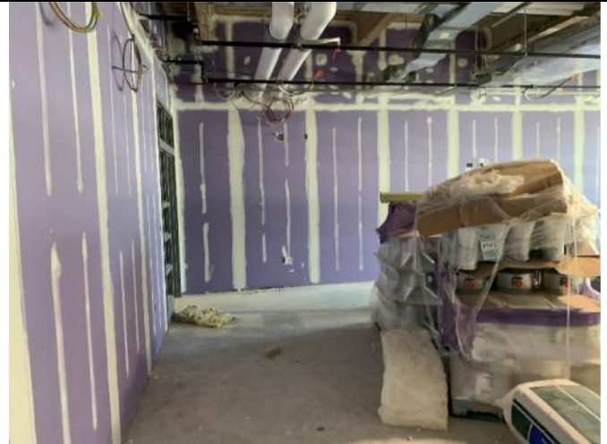
C2 1.25.21 Taping Gyp Board
