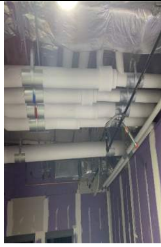
1/27 Pipe Insulation and Bathroom Rough In
